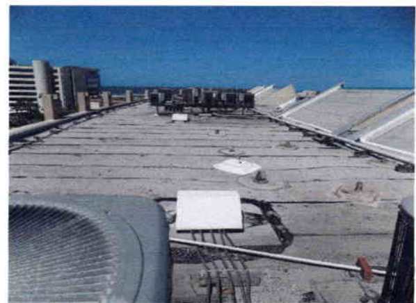
Modified Bitumen roofing
