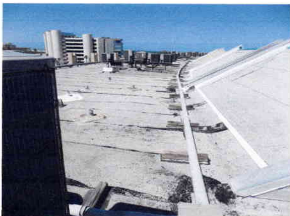
Modified Bitumen roof deck
