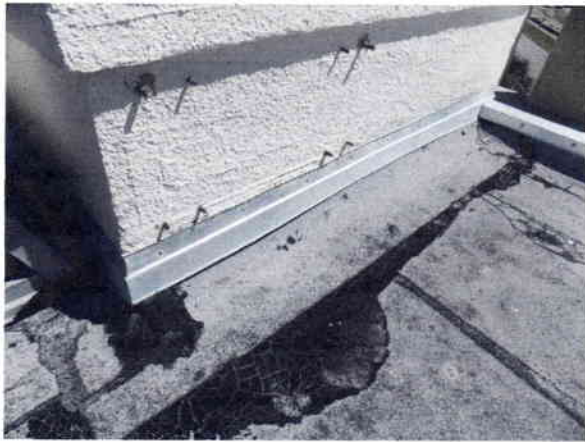
Mechanically fastened flashing
