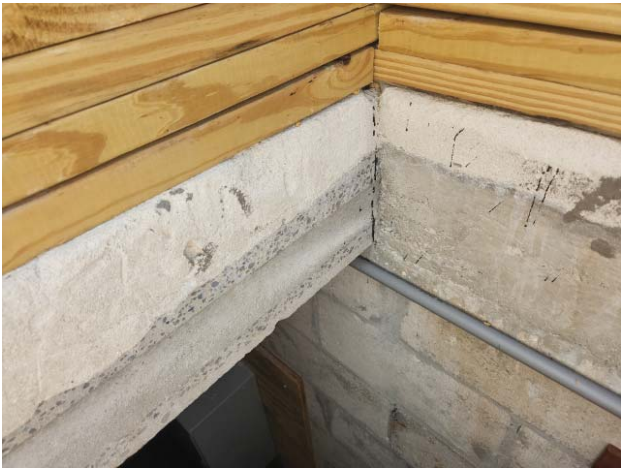
CONCRETE ROOF FDECK
