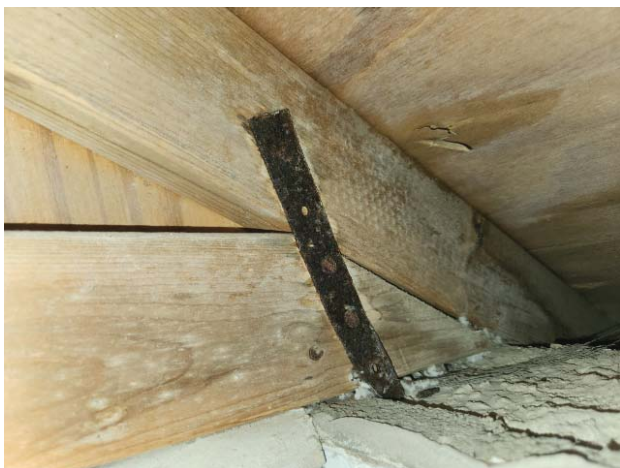
TRUSS CONNECTION
